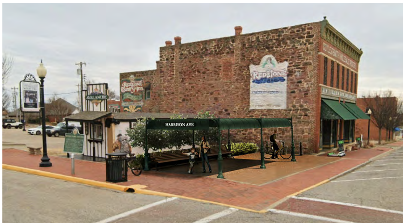
Figure 4: Pedestrians and cyclists enjoy the shelter, drawing attention to the red stone wall and historic mural to its south. Source: Peyton Kroh
