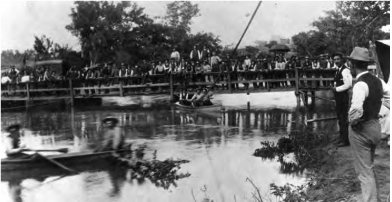
Historic photograph of a bridge over Cottonwood Creek. Year unknown. Source: Bob Chada
