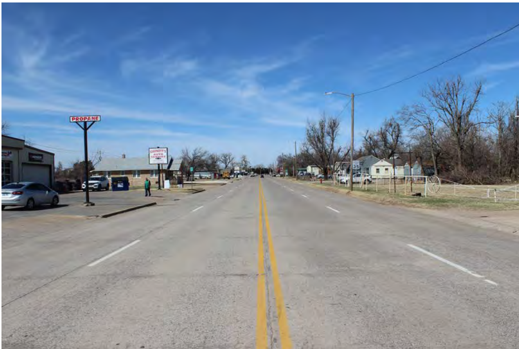
Typical view. Sunset Drive and Boynton Avenue.
