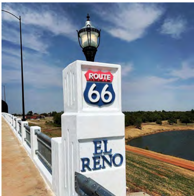
Newly renovated 66/81 bridge (Sandidge)
