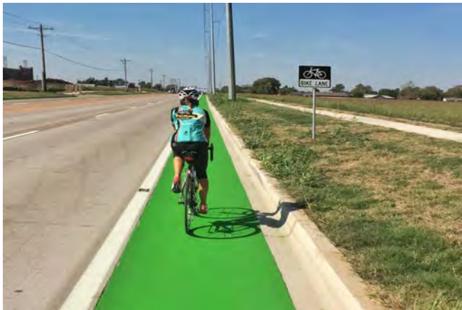
Bicycle lanes can offer a range of protection, from a simple striped lane to a physical separation. Norman.
