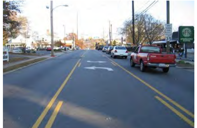
Center turn lanes help move more traffic with fewer lanes. North Carolina.
