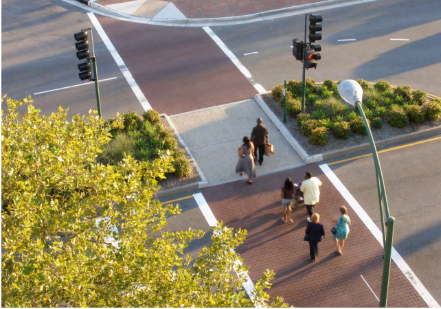
Figure 34. Median and Pedestrian Refuge Island
