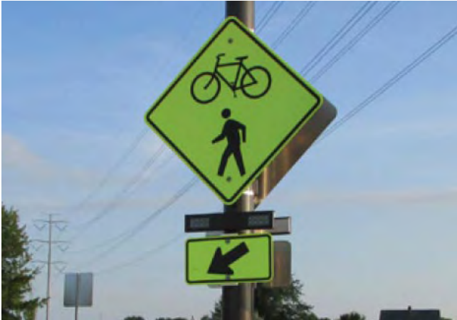
Figure 36. Rectangular Rapid Flashing Beacon
